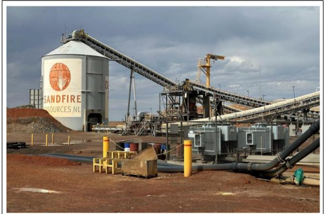
Figure 2: The DeGrussa Processing Plant
