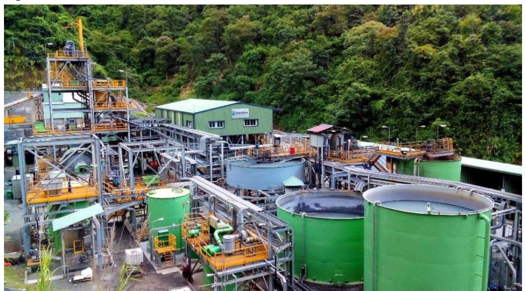
Figure 9: The Ban Phuc Process Plant
