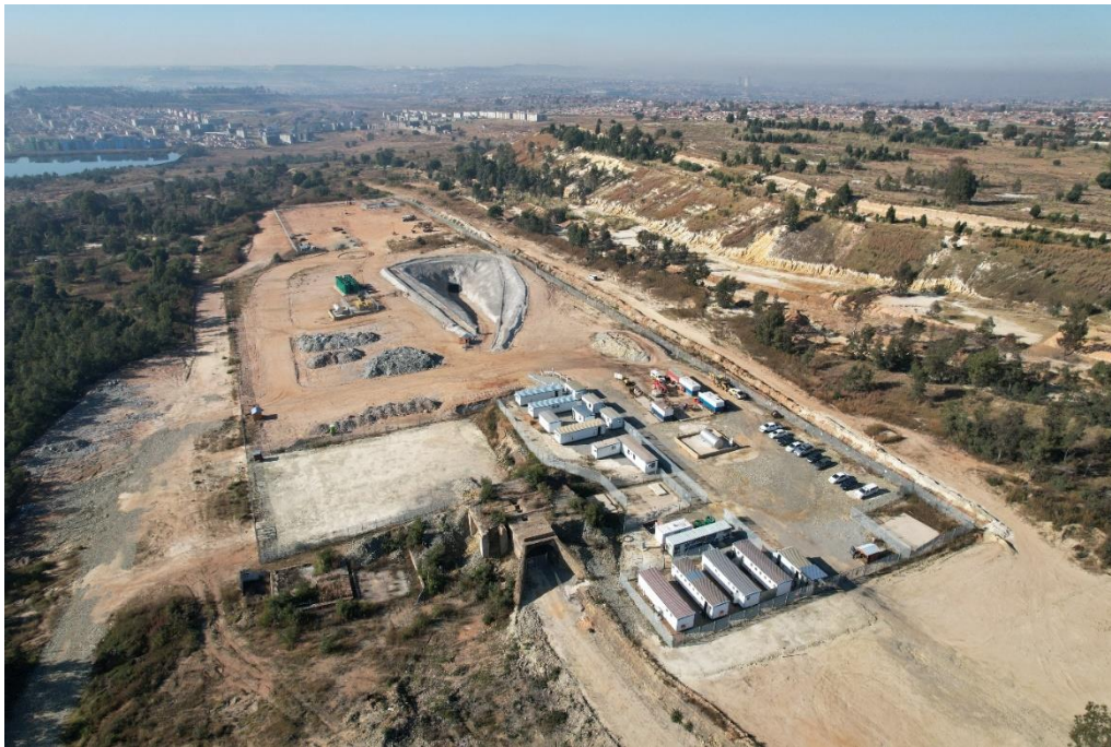
IMAGE 4: QALA SHALLOWS PROJECT PROGRESS
