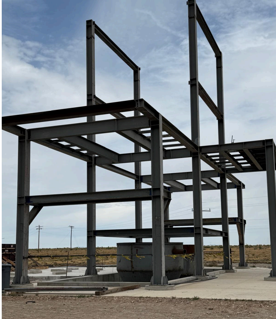
Fabricated Steel Components Being Fitted to Expanded Plant Structures.
