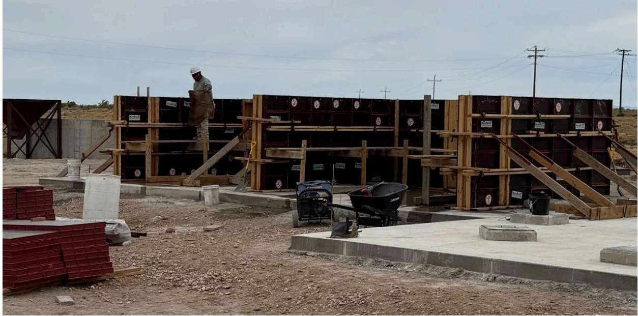
Concrete Pads and Structural Supports Being Erected
