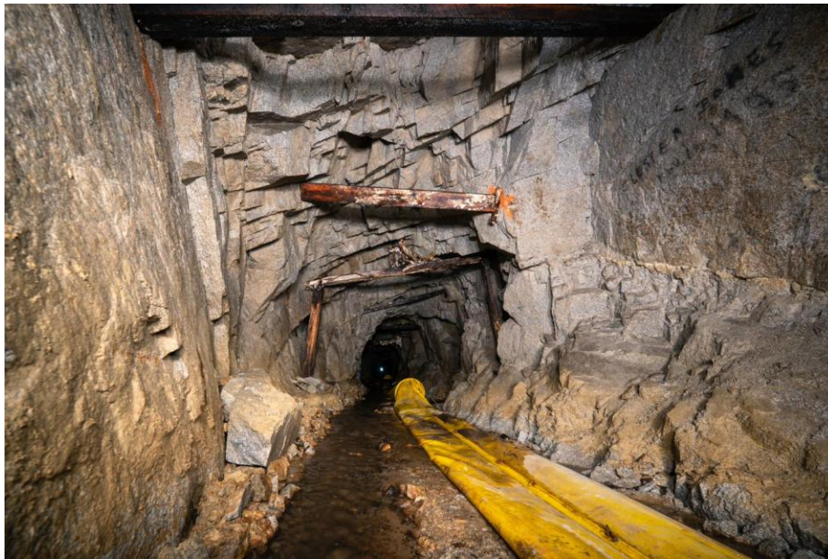
Figure E — Unity Tunnel in competent granitic ground beyond the timbered section. The tunnel remains open and walkable over substantial distances, with original timber sets and rail-era steel still in place.
