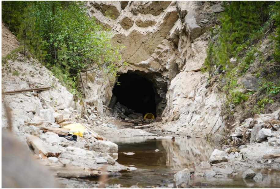
Figure C — The Unity adit at present. Water discharges from the portal, consistent with the gravity drainage function for which the tunnel was originally driven.
