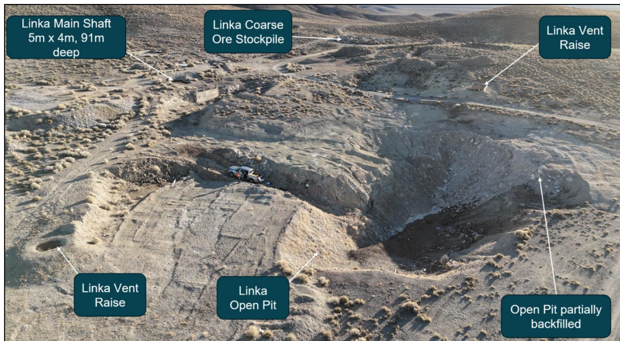
Figure 8: Photo looking south of the Linka Shaft, Vent Raises, Pit and Coarse Ore Stockpile.
