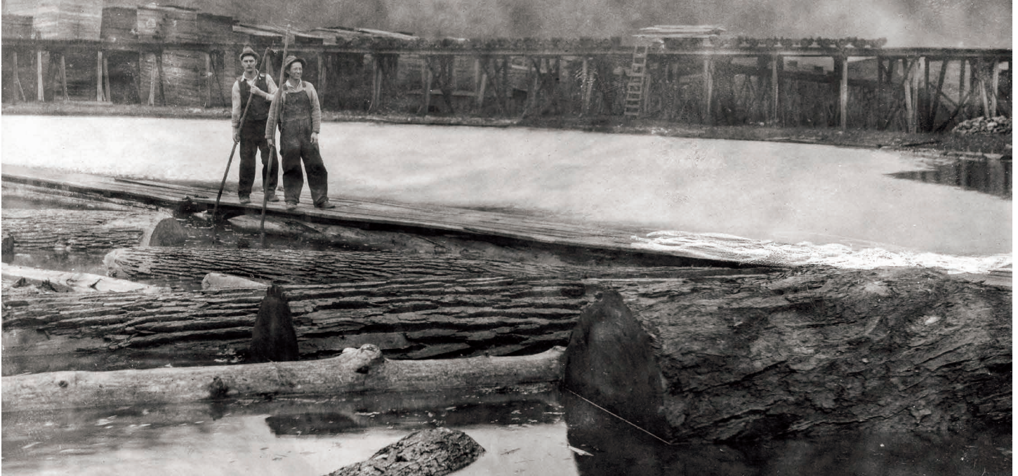
A railway spur and mill pond were built to allow floating log storage to prevent delivery interruption before going into the Pardee & Curtin mill in Bergoo, West Virginia. Logs stored in ponds had lower fire risks, washed off dirt that would normally have dulled saw blades, and also prevented the logs from splitting and drying out. Circa 1929.
