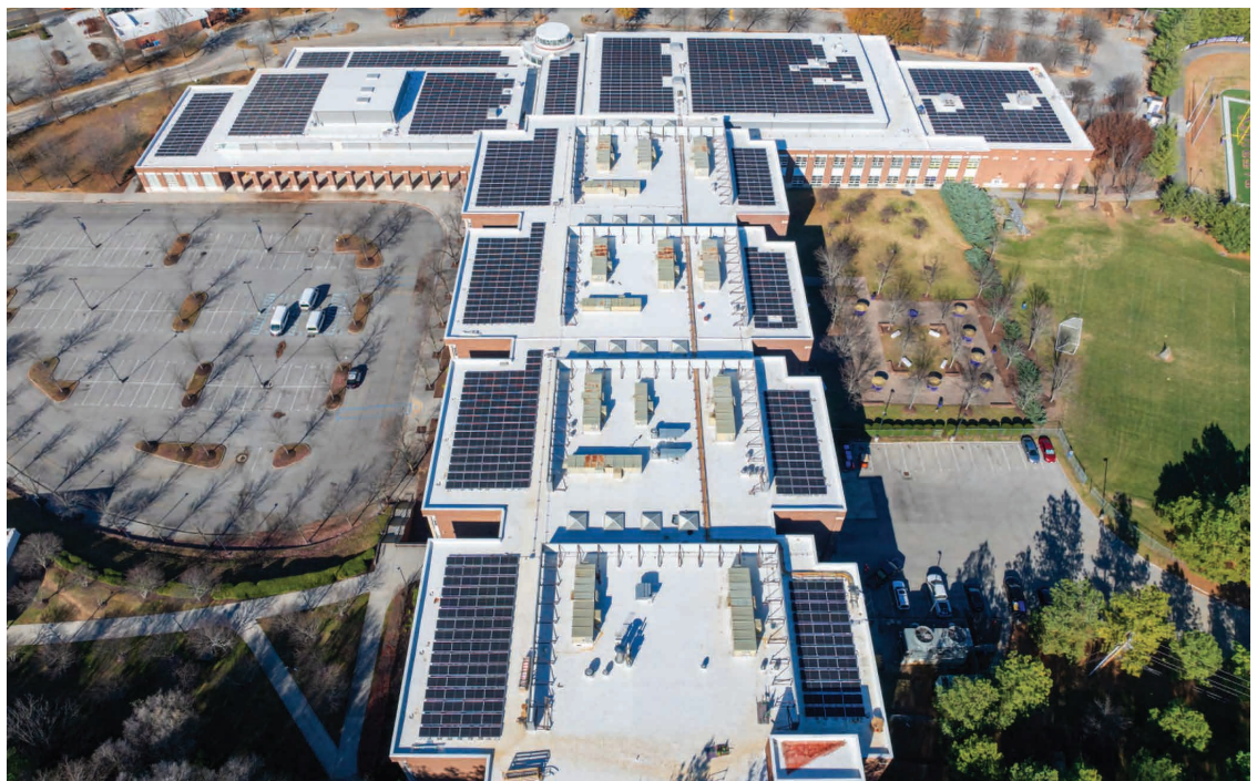
One of the Company's new solar photovoltaic rooftop systems located in Roanoke, Virginia.
