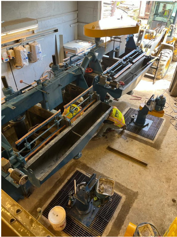
Figure 8a: Upgraded flotation cells being installed
