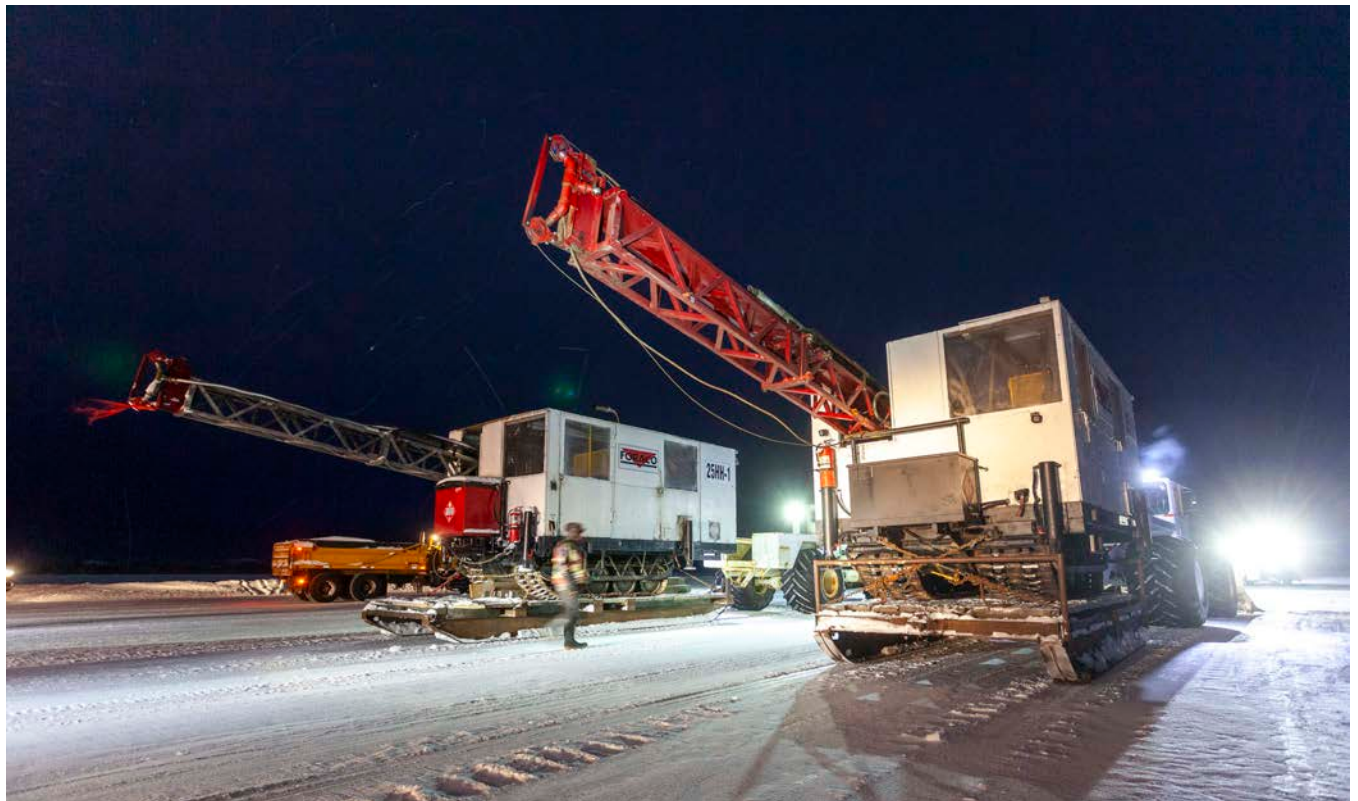
Figure 1: Mobilisation of Drill Rigs (February 2023)
