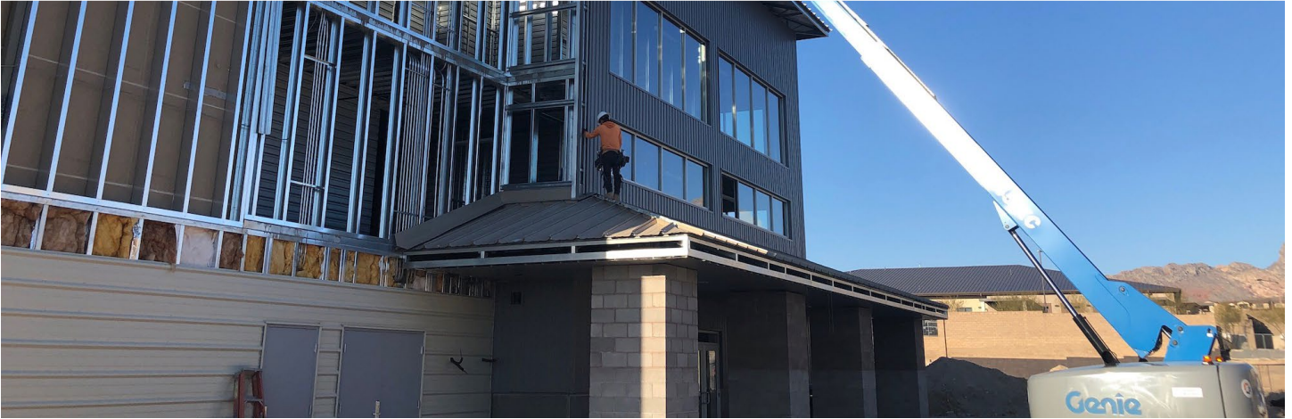
Redpoint Storage - Construction - Installing windows and siding on March 17, 2023
