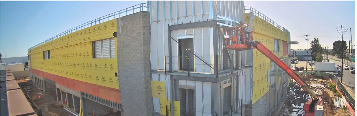
Santa Fe Springs Redevelopment - Installing siding on the new 3 story building on March 24, 2023
