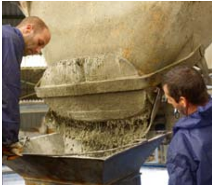
When concrete reinforced with Dramix® Green fibers is discharged, the mix retains its homogeneity
