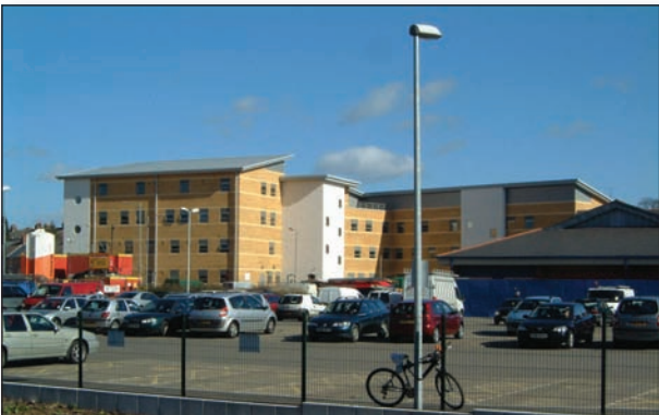
Prospect House Medical Centre Kettering, Northamptonshire Tenant(s): Two GP Practices and Pharmacy Date of completion: March 07 NIA: 39,500sqft. Cost: £11.4m
