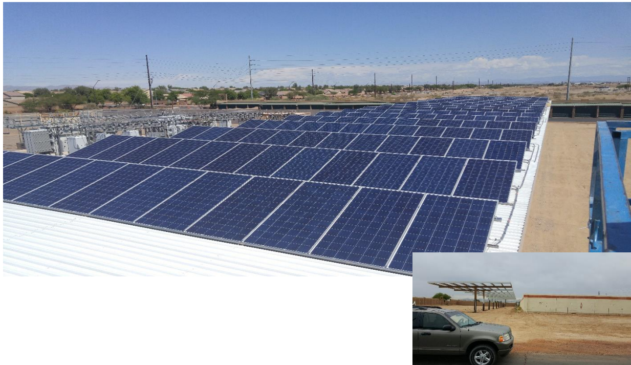
Under Construction in April 2016
