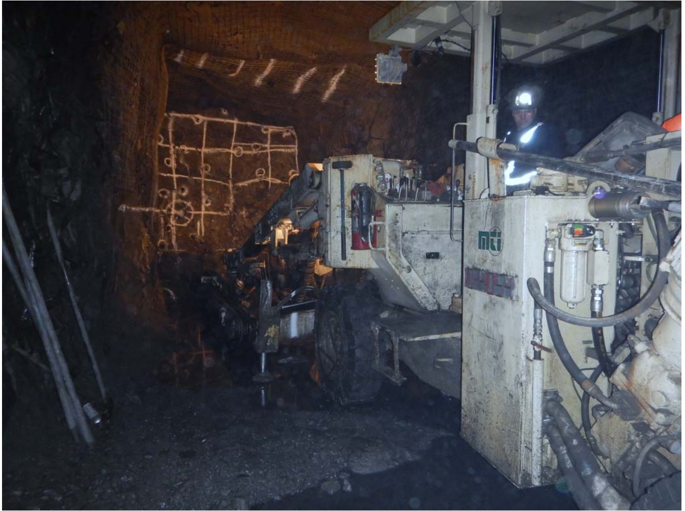
Figure 4: Underground development at Trevali's Caribou Mine
