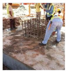
Thickener Center Column footing after concrete pouring.
