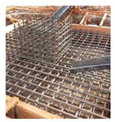
Thickener Center Column footing before concrete pouring.
