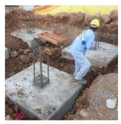
Stair Tower footing after concrete pouring.
