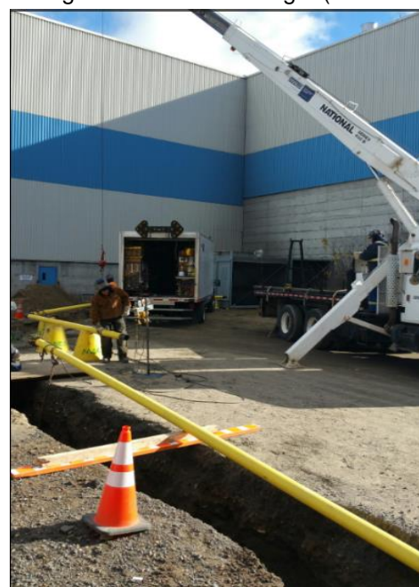
Phase 1 Plant equipment under installation and natural gas line being installed in Shawinigan(2016-11-04):
