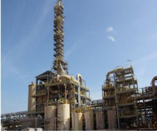
Waste Gas Treatment recovers acid and removes gaseous pollutants
