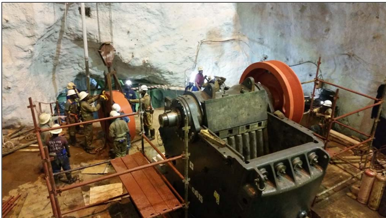
Figure 8: Installation of the two fly wheels (orange) onto the main frame of the new, primary rock crusher at Kipushi's 1,150-metre-level crusher station.
