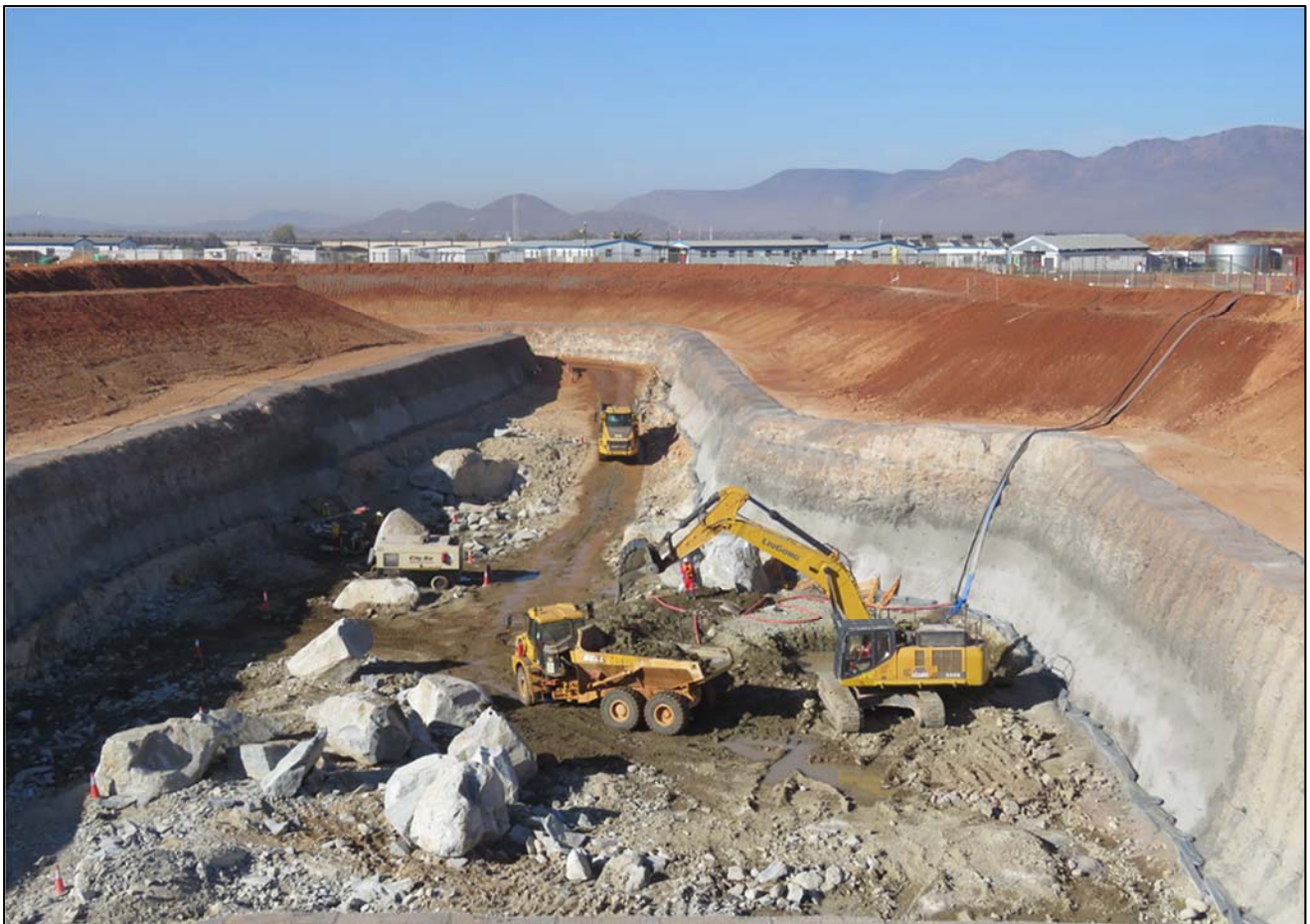
Figure 3: Removing blasted rock from the Shaft 2 box cut.
