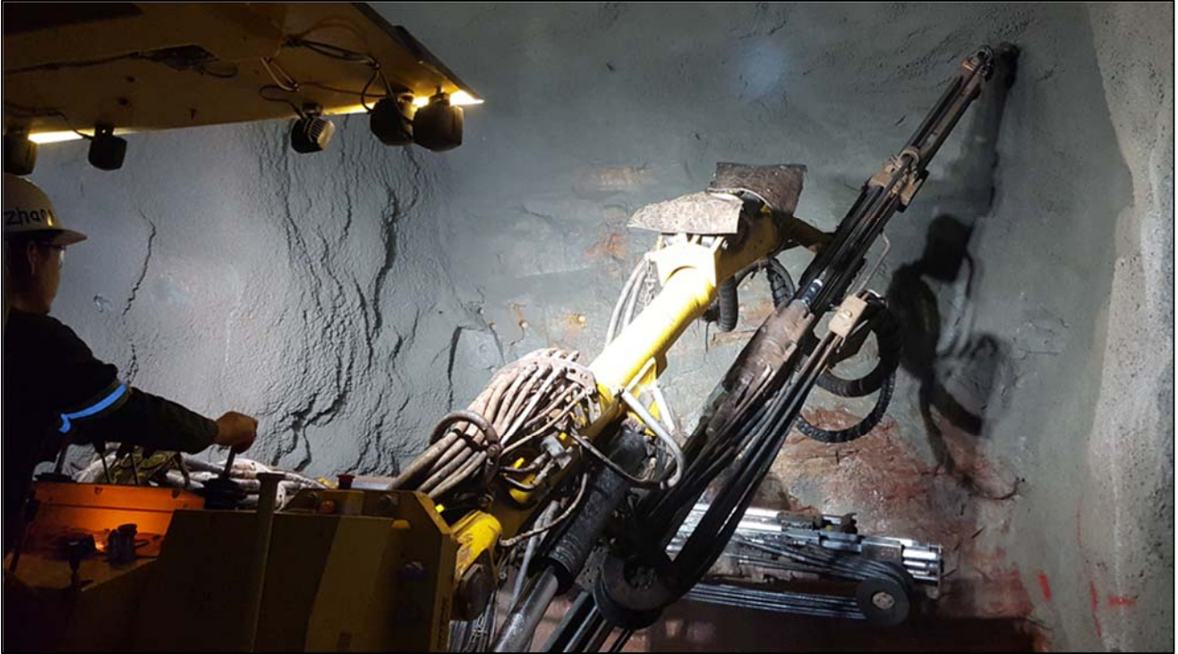
Figure 11: Drilling holes for explosives in preparation for a blast as part of ongoing excavation of the underground decline that will house the ore conveyor at Kakula.
