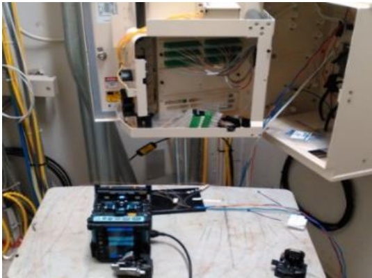
Inside Plant Fibre Splicing & Testing
