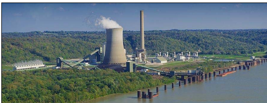
Figure 2: LG&E and KU's Trimble County Power Plant on the Ohio River (Note: Cooling tower is releasing water vapor)
