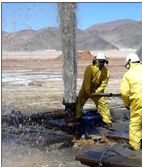
Figure 6.8 Airlift Effect at DRC-16
