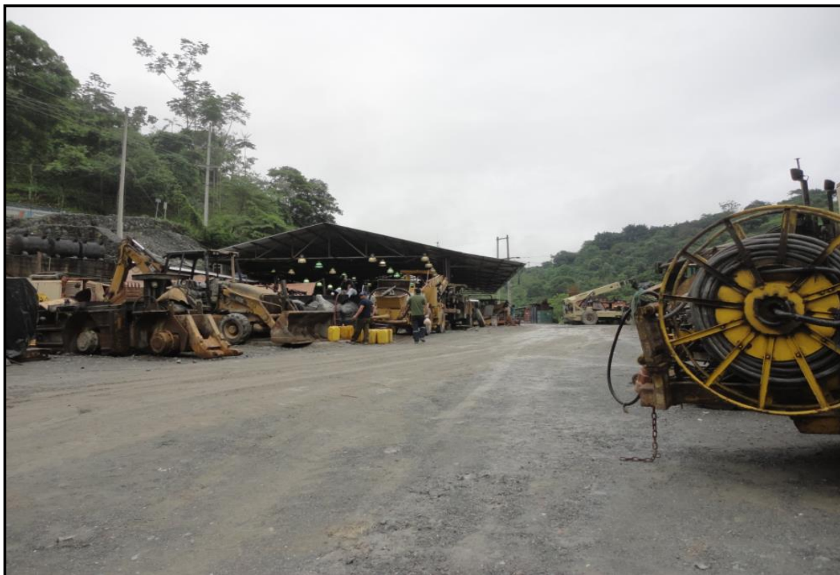
Figure 65: Entry to Underground Maintenance Facility.
