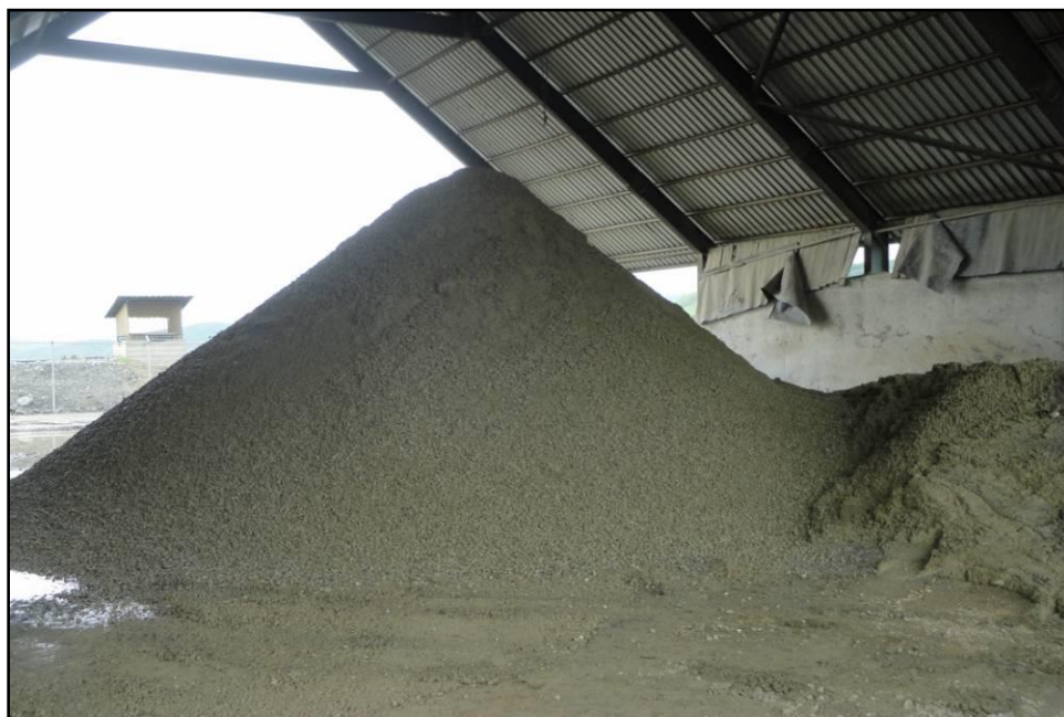
Figure 75: Fine Material Stockpile Silo.
