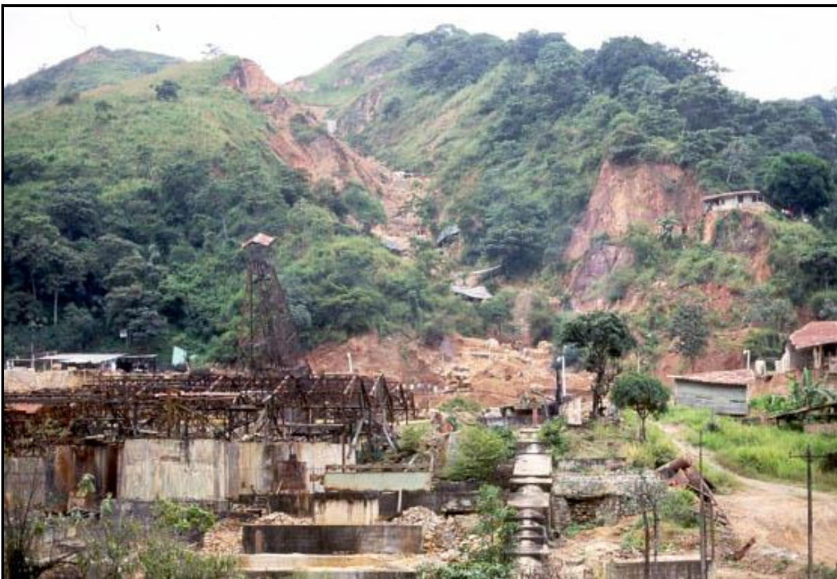
Figure 8: View of the Old SADC Vertical Shaft in Portovelo.
