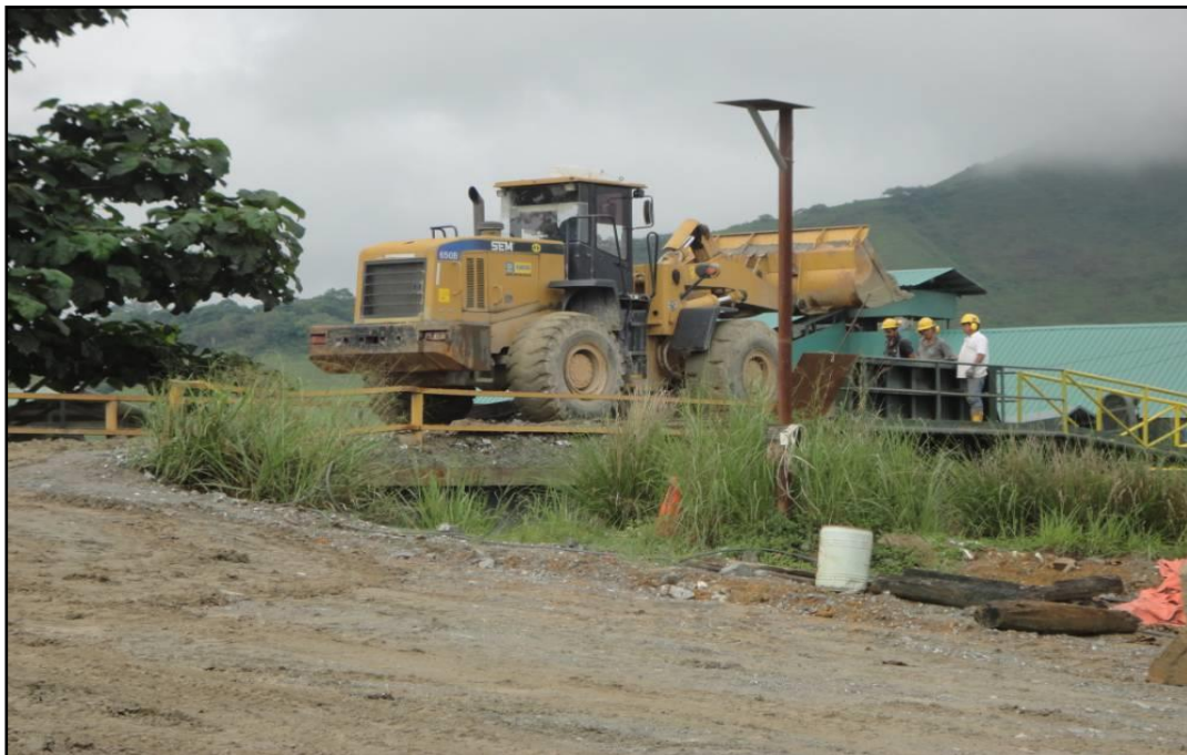
Figure 72: Front End Loader Discharging into Jaw Crusher Feed Hopper.
