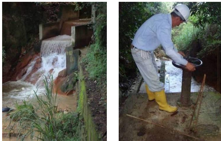
Figure 88: Water Damp System & Pressure Regulator.
