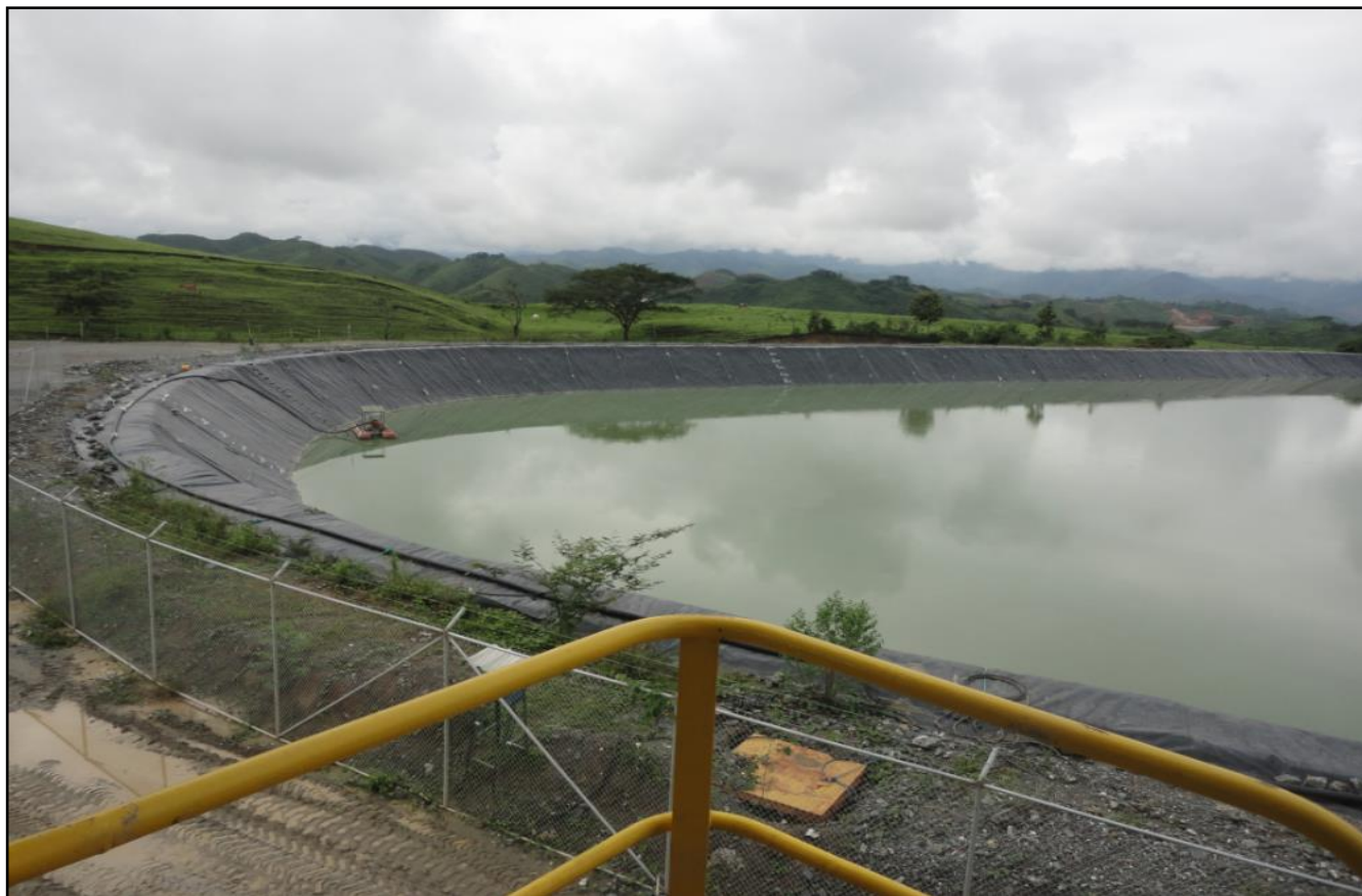
Figure 82: Processing Water Reclaim (Pond 2).
