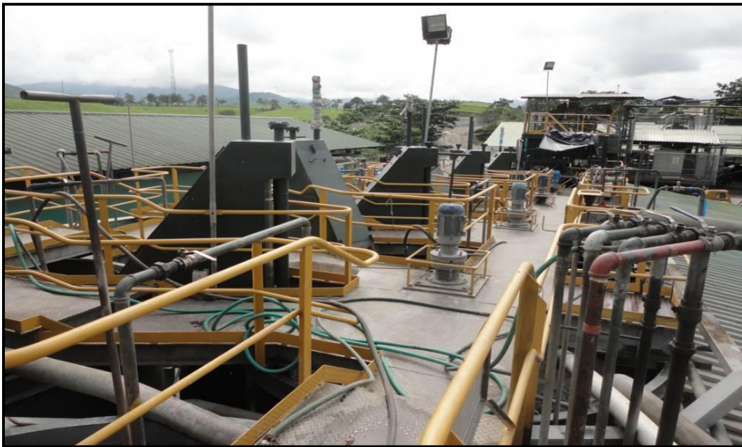
Figure 80: Platform of CIP Circuit Tanks.
