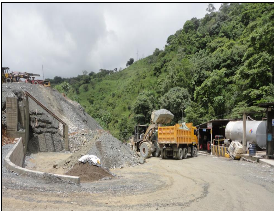
Figure 64: Underground Material Loading into 30 t Dump Trucks.
