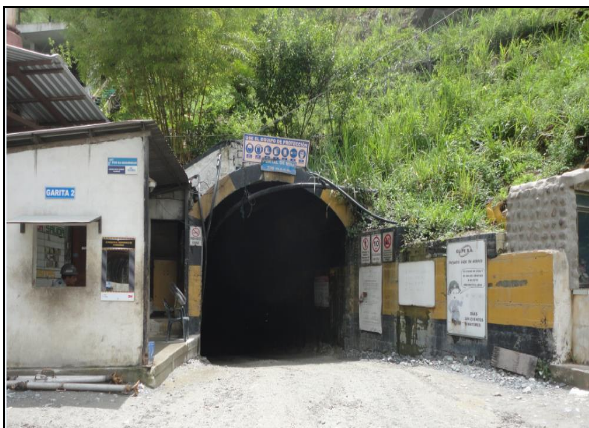
Figure 63: Portal for Underground Access.
